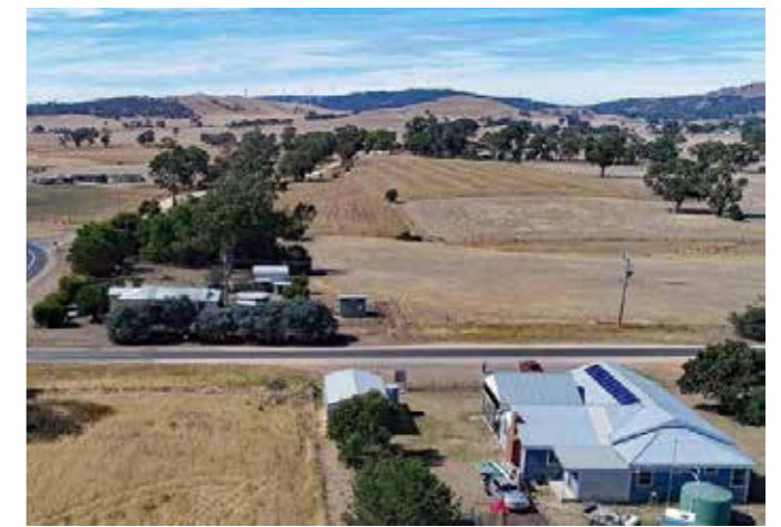
Crowlands Hall rooftop solar installation
